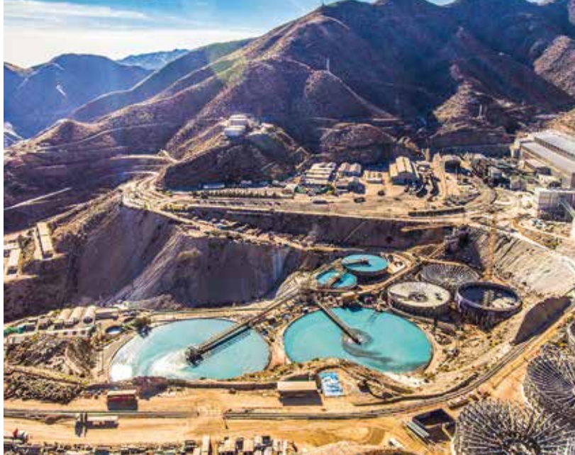
© Southern Perú Copper Corporation
